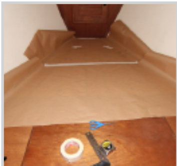
9 - Lay out 2nd Layer of paper. From one side to other & Tape to the 1st Layer of paper.
