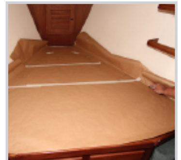
12 - Lay out 3rd Row of Paper and Overlap Around edges. Tape down to the 2nd Row of Paper.
